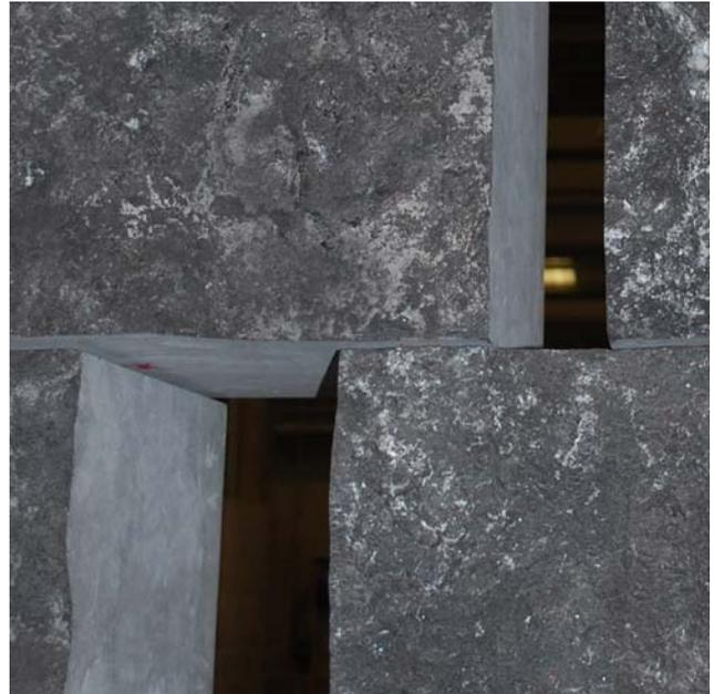
The wall is necessarily massive. Though capable of being an inertia wall the individual blocks are dowelled together to form a continuous framework. No opening at the lower level is greater than 100mm. The “rear” and sides of the stones have a sawn finish revealing the fossils buried in the stone. Though unpolished the stone reveals this secret when wet.
